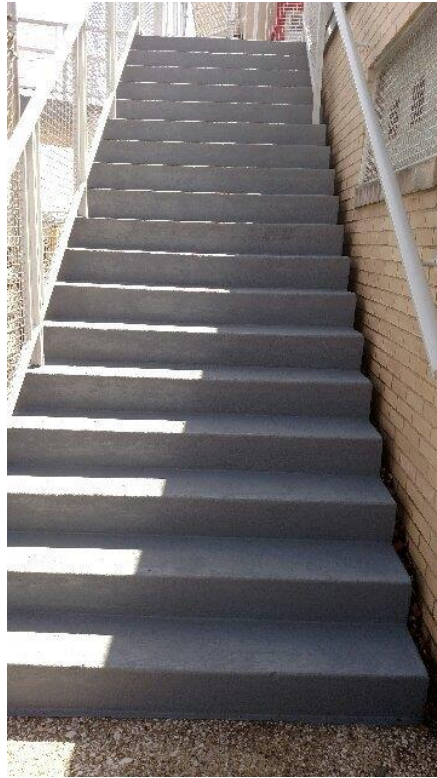
Non-slip, rubberized Walking Surfaces
